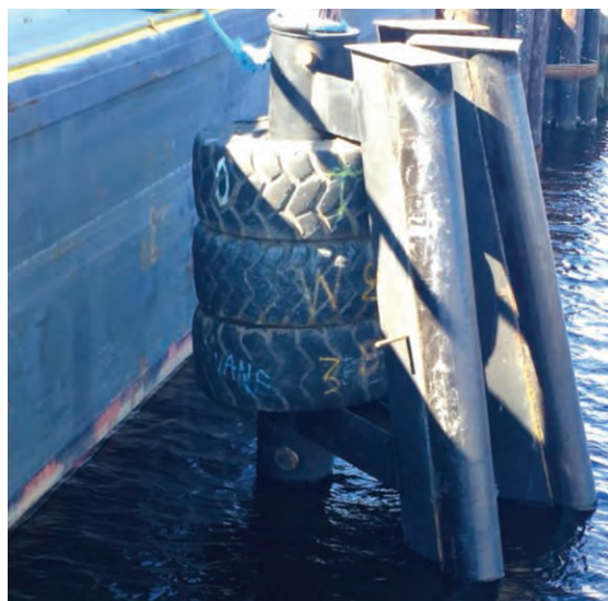
General Ship Repair has produced prefabricated steel pipe pile fender units for Vane piers.
